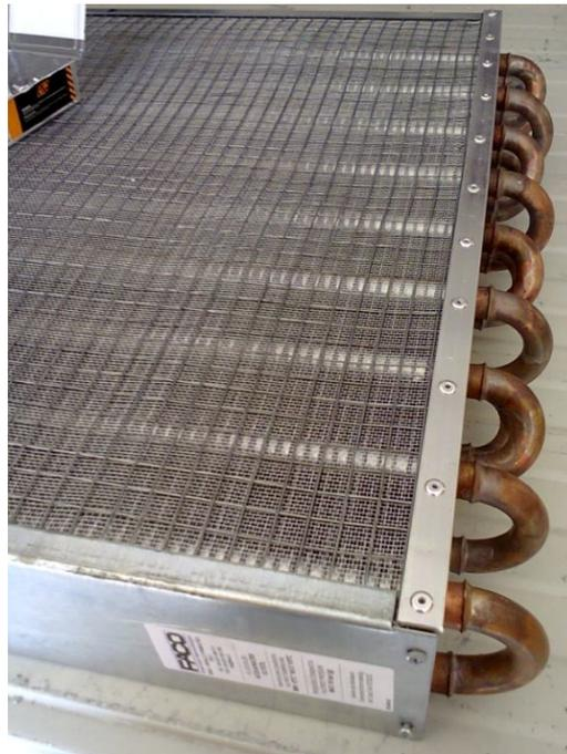
**Figure 5: Packed adsorption bed**
